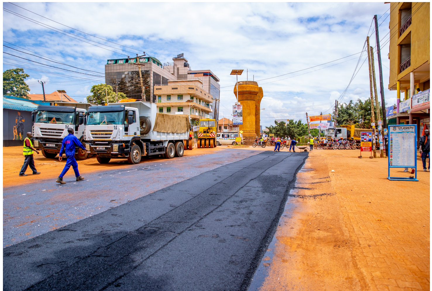
Laying of Asphalt on Kabaka Anjagala Road to Lugaga Cathedral junction
