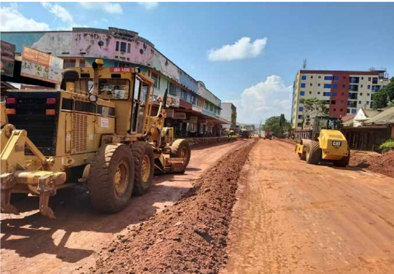
PROCESSING OF ROAD SUB-BASE LAYER
