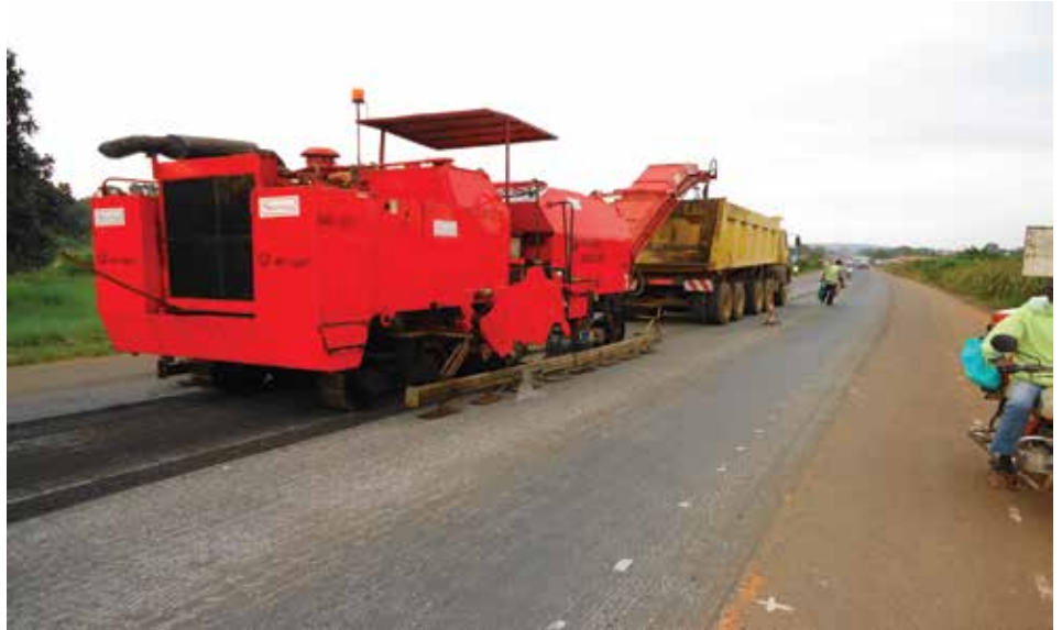
MILLING OPERATION
