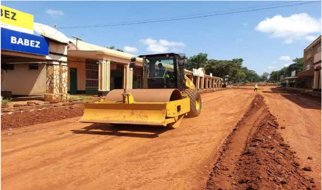
PROCESSING OF ROAD SUB-BASE LAYER
